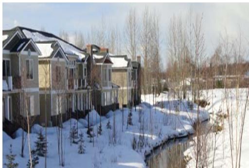
Photo 31: Local Creek Restoration – Greenway-supported Development
