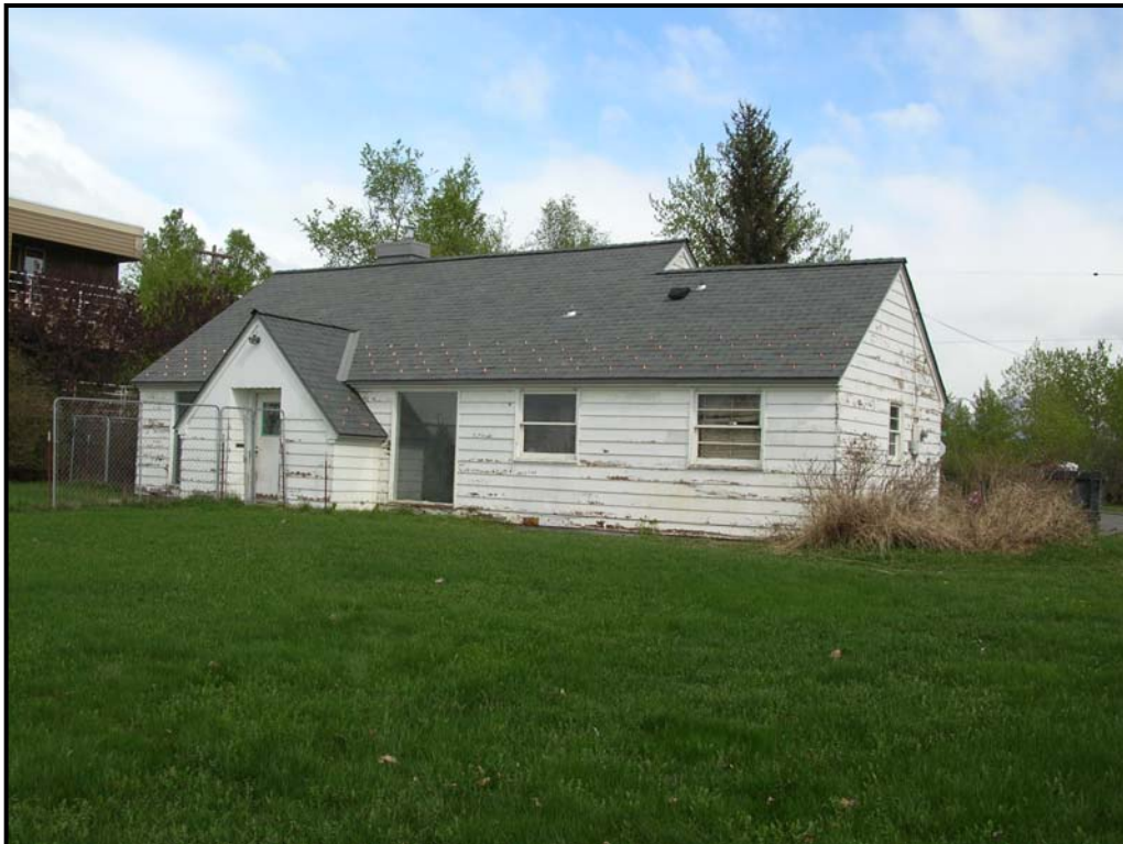
Below: 800 Delaney Street is shown here from the bluff edge in 2005 before undergoing restoration.
