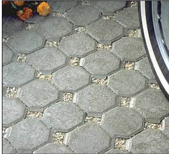
Figure 7 – Open-Jointed Paving Block
