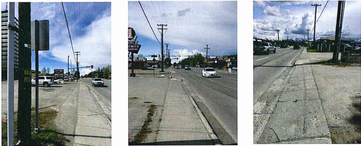
Figure 4: Dense Driveways, Non-ADA Compliant Cross Slopes, and Other Issues
