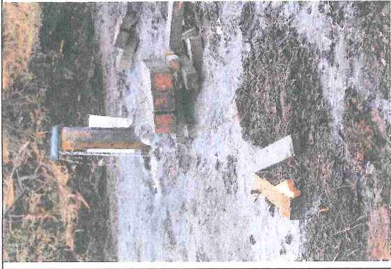
Wellhead leaking 1.3 gallons per minute Developer knew it was leaking. Over 250,000 gallons of water released.
