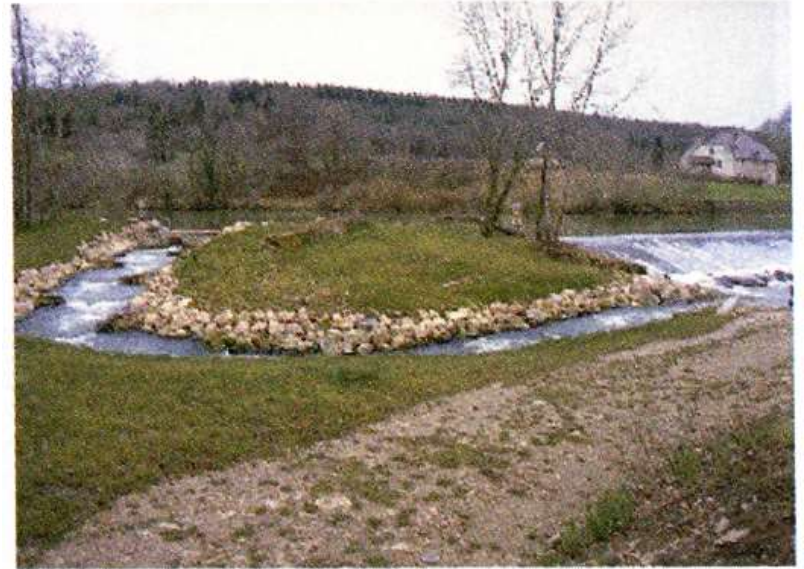
Photo 14: General view of the natural bypass channel at
