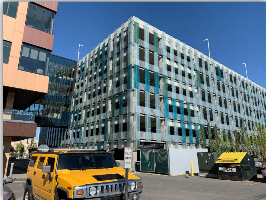
A new garage on ANTHC's campus
