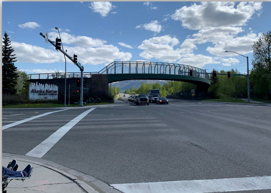
Tudor Rd. pedestrian and bicycle overpass
