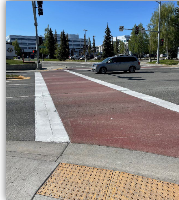
Truncated domes and high visibility crosswalks at UAA Dr. and Providence Dr.
