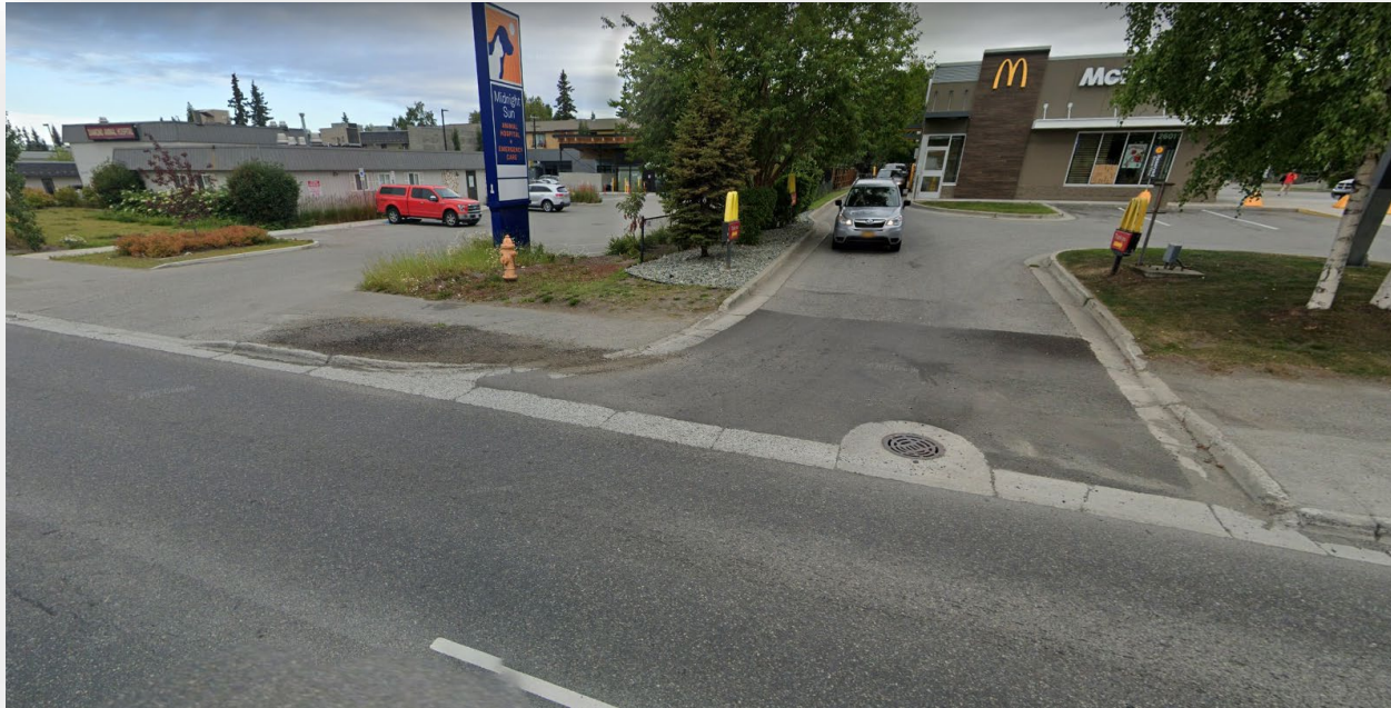
Missing crosswalks and truncated domes along Tudor Rd. limit ADA access and pedestrian visibility
