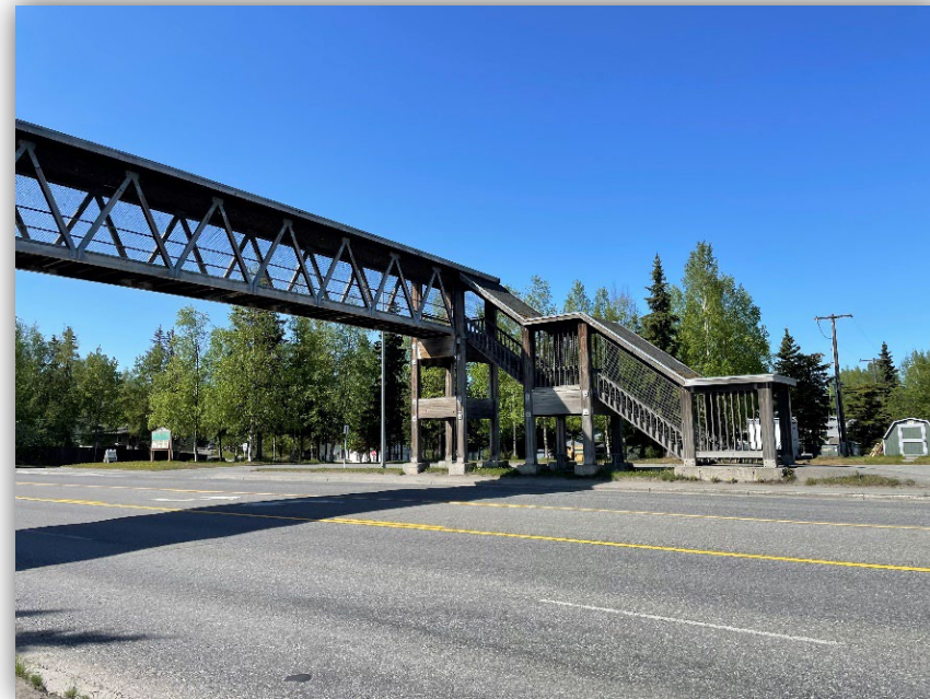
Lake Otis Pkwy. pedestrian overpass
