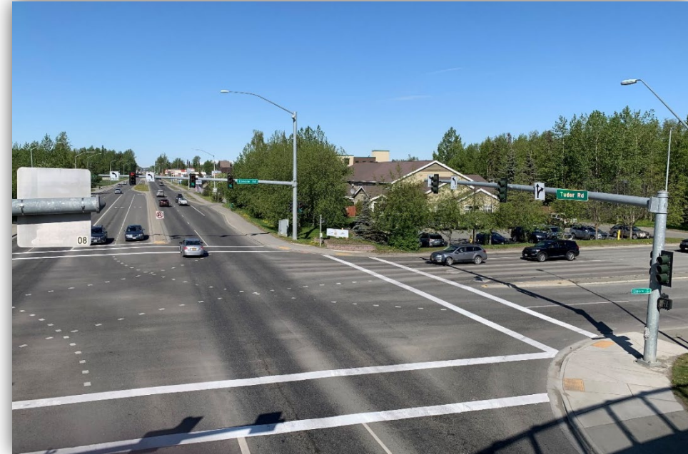
Double left turn pockets provide additional vehicle throughput into UMED, but increase crossing distances
