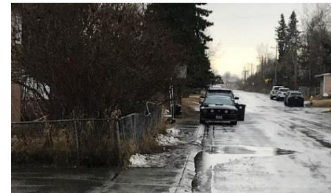
Parked car and remnants of plowed snow on a cracked, broken sidewalk.
