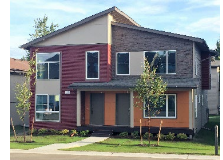
Good site access for pedestrians.
