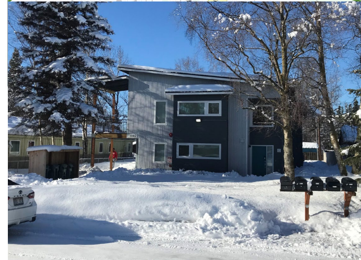
Two-story four plex at 3602 Oregon Drive, with 2 units on top floor and 2 units on first floor. View from street. Lot size is 9,800 sf. R-3 zone allows up to a six-plex on 9,000 sf lots.
