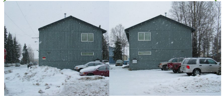
Multifamily site with a pair of four-plex townhouse style buildings at 9 th Avenue and Medfra Street. Observed peak period parking utilization was 5-7 parked cars, including cars parked on-street on curb along the property's frontages.
