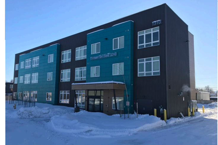
Three-story multifamily apartment frontage on W. 32 nd Avenue near Spenard Road.
