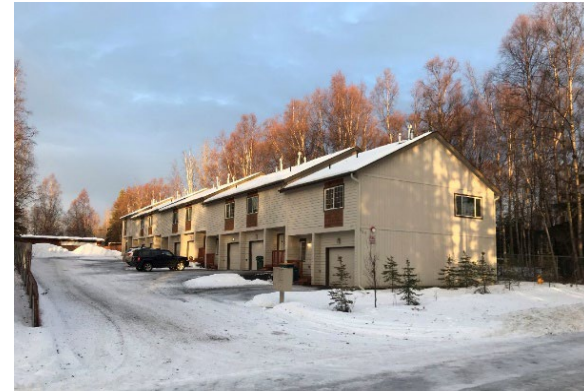
Large driveway area into multi-family housing inconsistent with surrounding single-family driveways.
