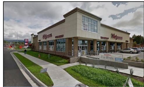
A pedestrian-supportive street frontage.
