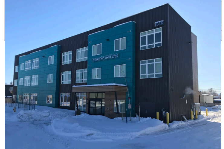
Cook Inlet Housing Authority (CIHA) three-story multifamily apartment fronting on W. 32 nd Avenue near Spenard Road.
