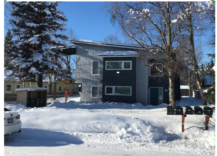
Two-story four plex at 3602 Oregon Drive, with 2 units on top floor and 2 units on first floor. View from street. Lot size is 9,800 sf. R-3 zone allows up to a six-plex on 9,000 sf lots.
