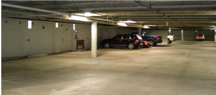
Parking oversupplied due to parking minimums.
