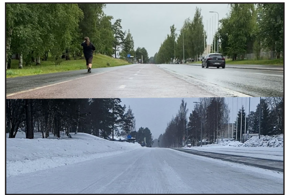
Pedestrian path of 8'4", cycleway of 13'4", and total width of 21'8". Since the total width is without curbs to allow the snowplough to treat the entire surface. Winter clearing produces a level surface of snow.
