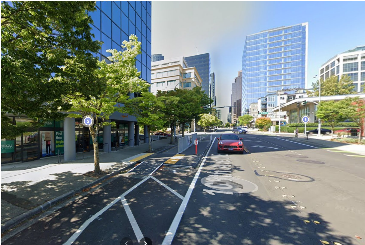
Figure 14. Boarding Island Constructed with Zicla© Blocks in Bellevue, WA (Source Google Maps)
