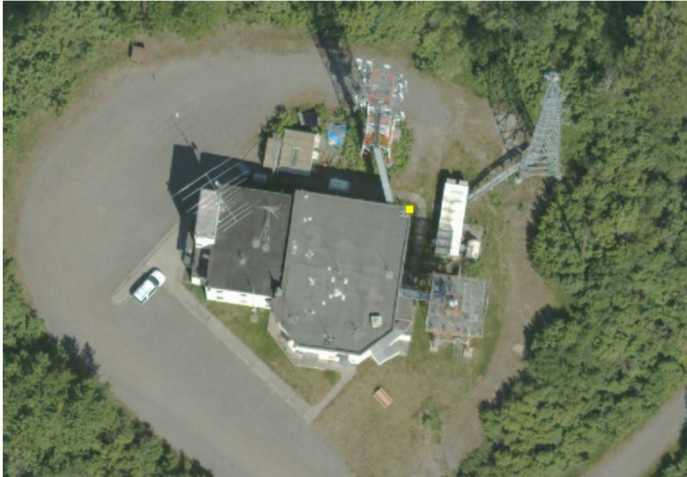
Figure 1. Aerial view of Building 16322 and associated structures.
