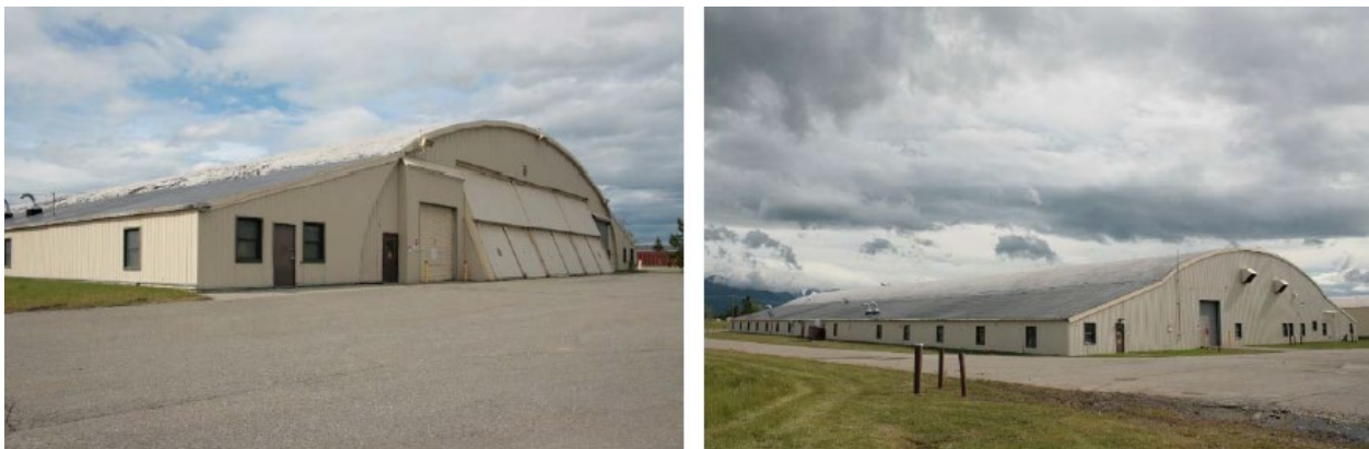
Figure 3. Building 8326 exterior – view of McKee cantilever doors and administrative wings.
