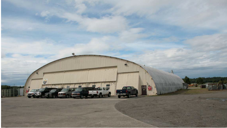
Figure 2. Building 7301 exterior – view of barrel roof and McKee cantilever doors.
