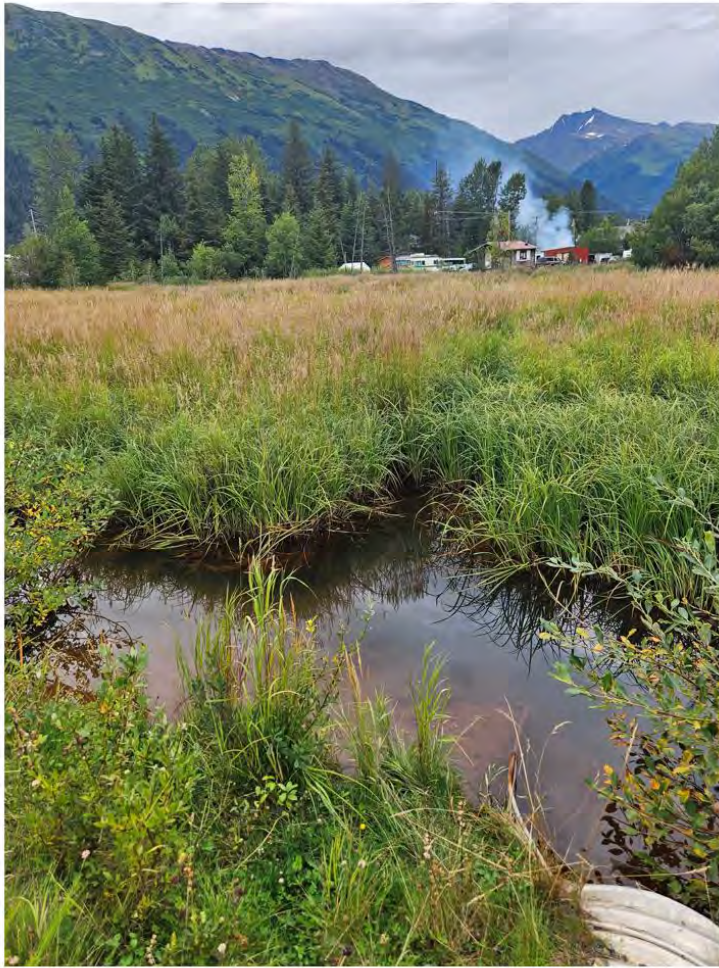
North end of Culvert
