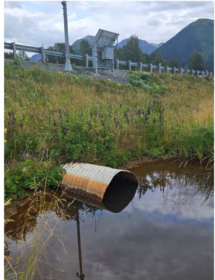
South end of Culvert
