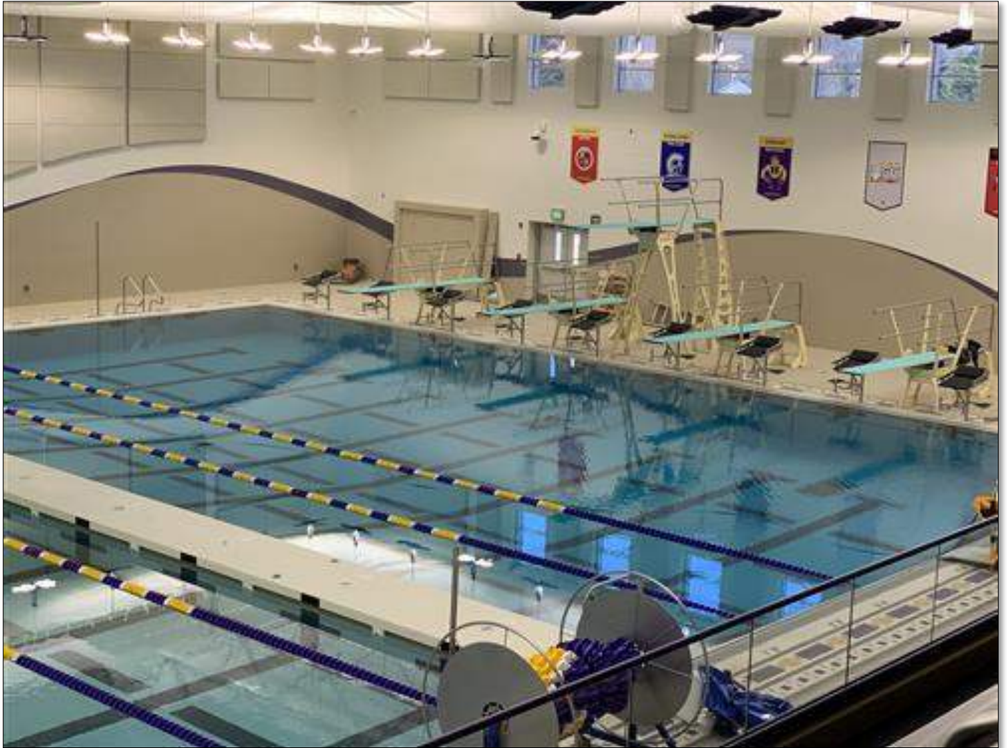
Figure 20- More stilt stands- note that stilt stands make the hand railings static, and interfere more with swim starts. Yet this installation is still legal and works!
