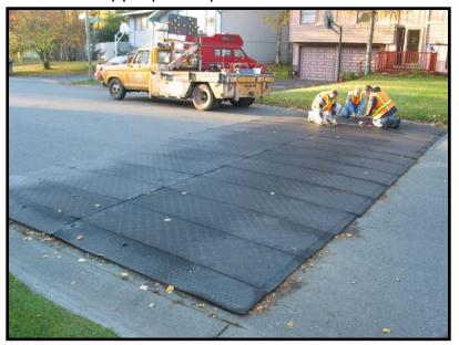
Temporary speed humps are 14 feet in length and varies to a maximum of 3 inches in height.
