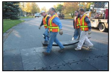
Many physical constraints dictate the placement of temporary speed humps. Compared with permanent speed humps, more latitude exists for the use of temporary speed humps due to their placement during summer months only. Installation of temporary speed humps begins in May each year and removal must take place prior to snowfall; therefore, all of the humps must be removed by October 15<sup>th</sup> each year. The following is a list of placement constraints:
