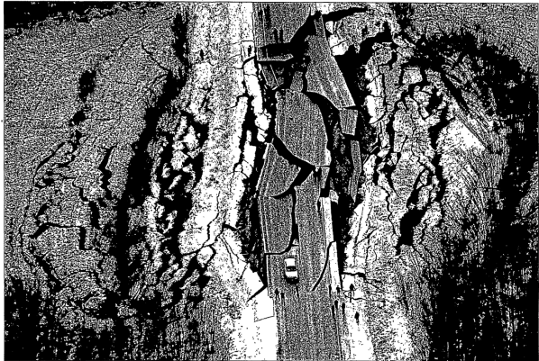
Vine Road, southwest of Wasilla, was heavily damaged by Friday's 7.0 earthquake.
