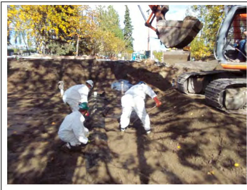
Photo 14: Facing north, BCX completed the VES installation by shoveling pea gravel on the horizontal pipe, closing geotextile, and placing soil over the assembly to prevent the geotextile from opening. (9/13/2011)
