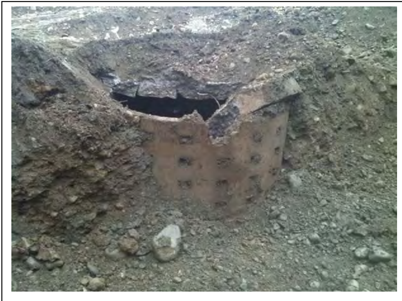
Photo 5: The dry well consisted of a 4-foot diameter perforated concrete pipe. (9/6/2011)
