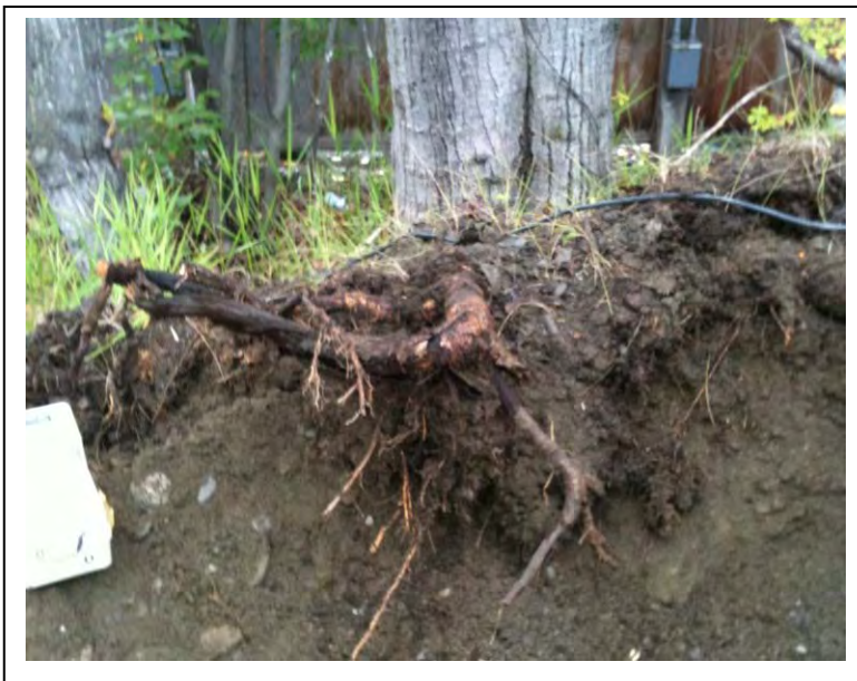
Photo 20: Facing south, the root wad on the south edge of the excavation prior to removal. (9/2/2011)
