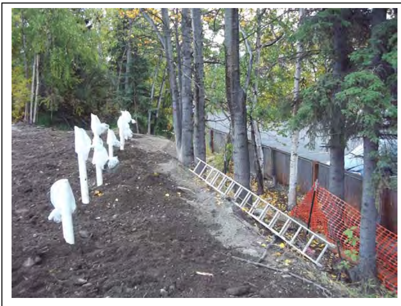
Photo 18: Facing east, the south VES risers can be seen. To the right (south) of the risers, the property slopes down, and trees and a fence are present. (9/15/2011)
