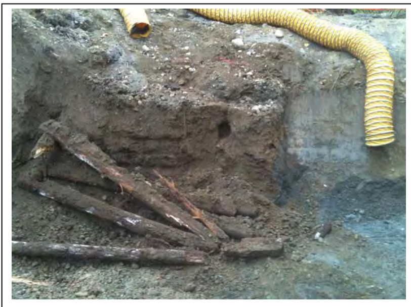
Photo 6: Facing east, the exposed portions of the log crib are shown. (9/6/2011)
